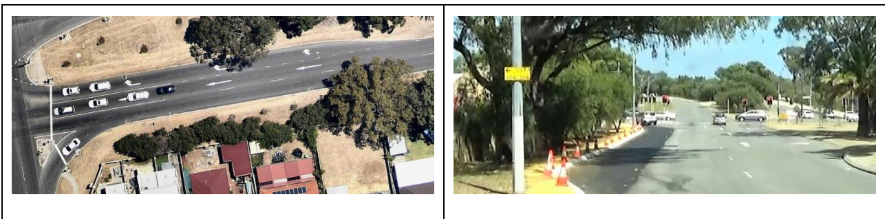
Nearmap aerial showing no left turn auxiliary lane and site visit showing recently constructed lane
